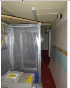
Soft strip & asbestos removal to East Wing
